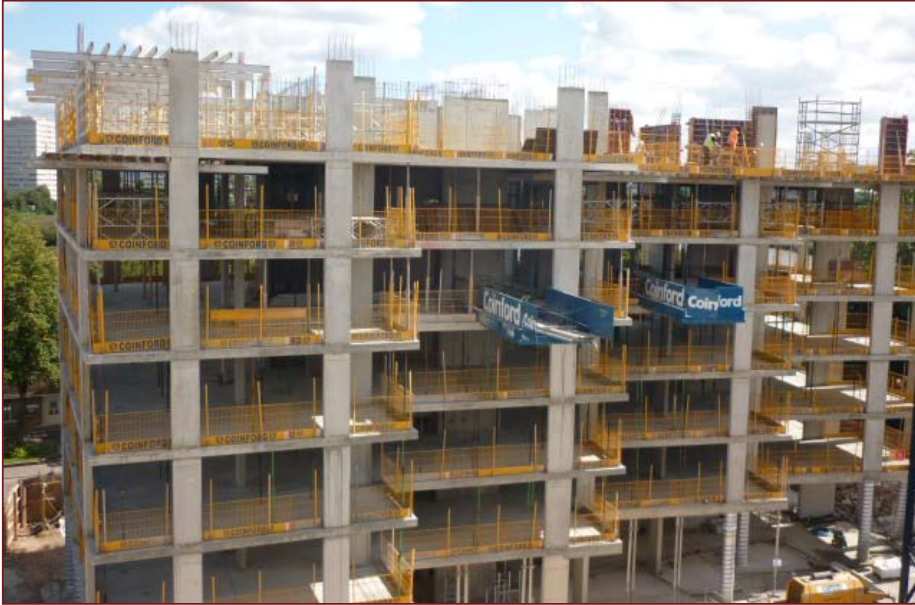
New homes under construction on the Old School Site
