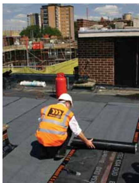
Inspecting new roofing at the Mapledene Estate in Queensbridge
