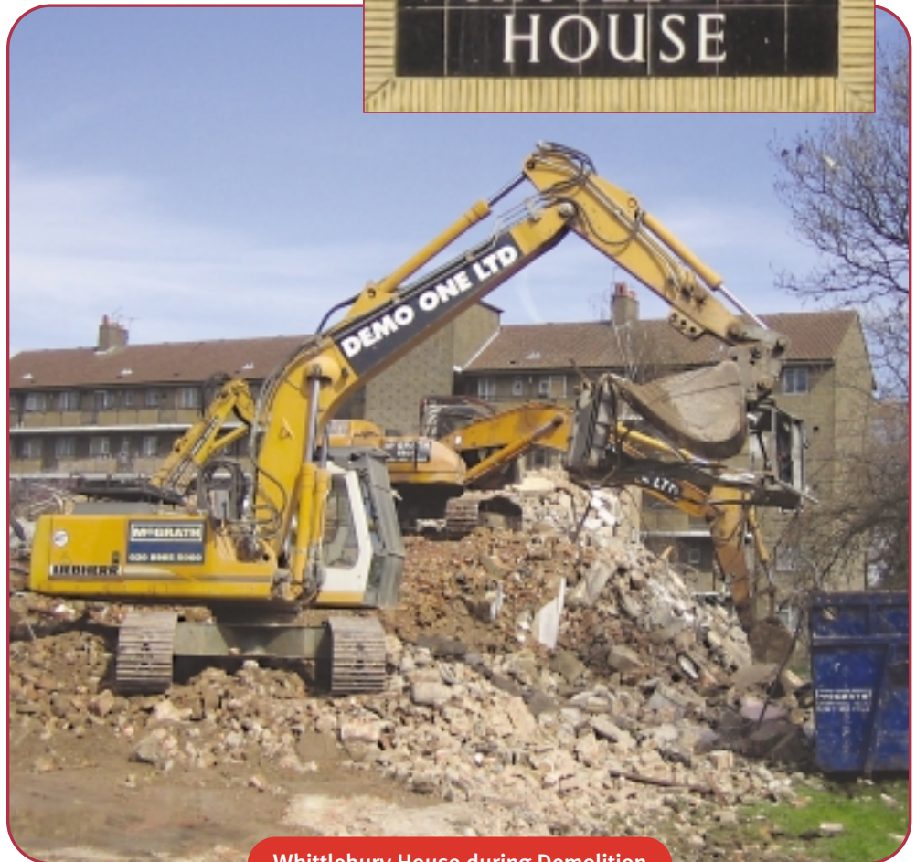
Whittlebury House during Demolition
