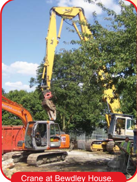
Crane at Bewdley House.
