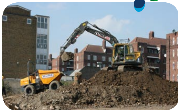
Above: Demolition work on the Old School Site.
